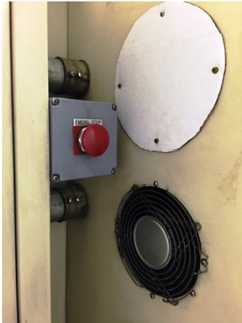
Check for dead and missing fans
