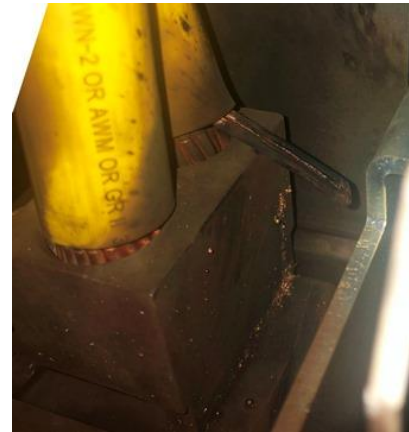
Wire whisker short circuit
