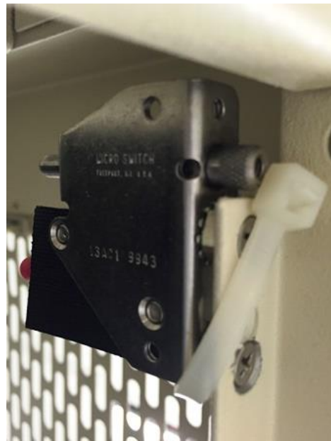
Door interlock should not be easily defeated
