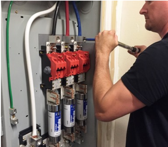
Good: wiring terminals torqued to spec
