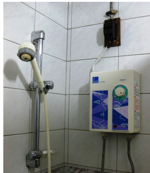
Electric water heater in a shower stall
