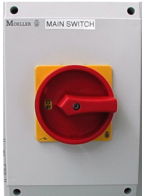
Disconnect can be red & yellow rotary switch
