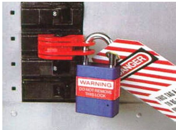
Cal-OSHA permits temporary clips for LOTO. NEC 110.25 states that portable locking mechanisms intended for temporary application are not acceptable for LOTO.
