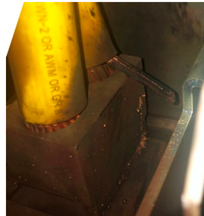
Wire whisker short circuit
