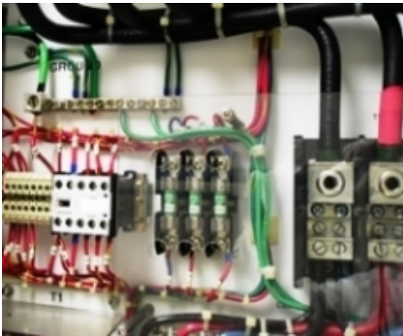
Neat and safe wiring with touchproof guard
