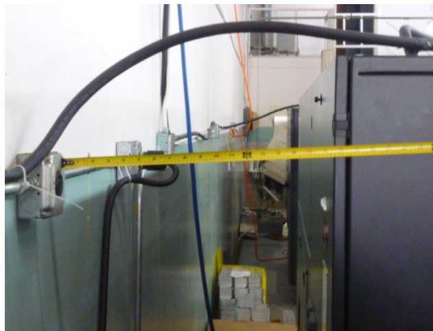
Inadequate clearance – must be 36 inches
