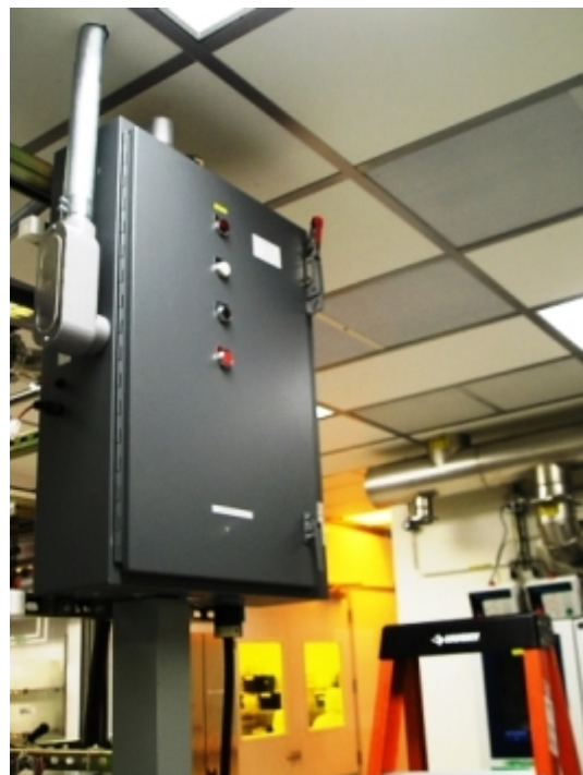
This disconnect switch is too high. It should be "readily accessible" and not require a ladder.
