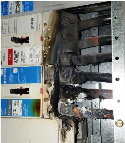
Loose terminals, then oxidation, then burn-out
